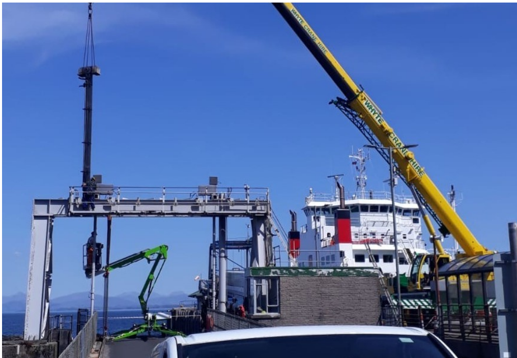
Replacing hydraulic cylinder - Craignure
